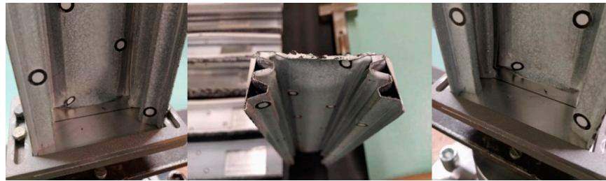
Figure 8. Columns after performed tests.
