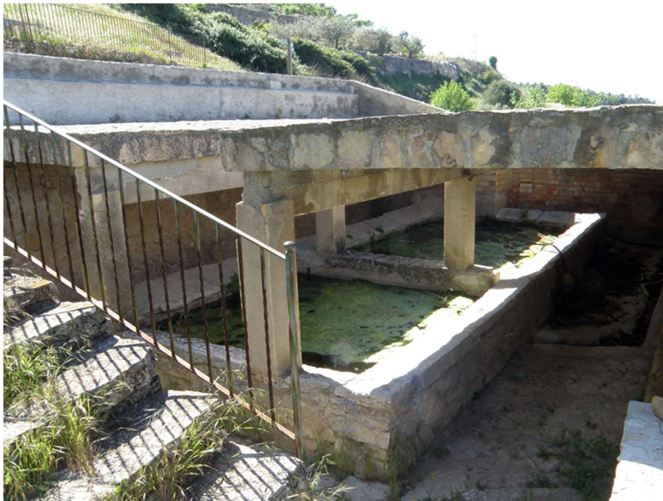
Figure 8. Wash place next to the Font Vella spring (la Figuera). This was restored in recent times with the repairs of their masonry wash basins and stone scrubbing decks.
