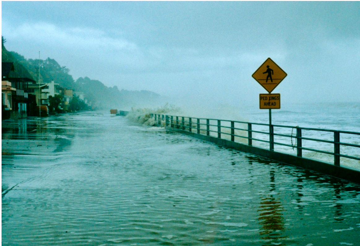
Figure 14. Flooding of Beach Drive in Rio Del Mar along the northern Monterey Bay shoreline during the 1983 El Niño.
