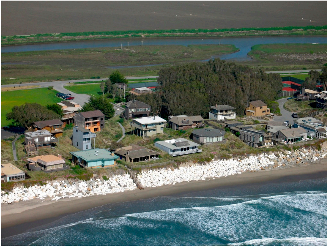
Figure 11. Rip rap revetment placed against eroded dune face at Pajaro Dunes (Photo April 2006).
