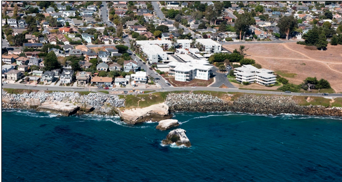
Figure 4. About half of the three miles of West Cliff Drive in the city of Santa Cruz has been armored with rip rap. Does this rock constitute a living shoreline? (Kenneth and Gabrielle Adelman, California Coastal Records Project, Californiacoastline.org ).
