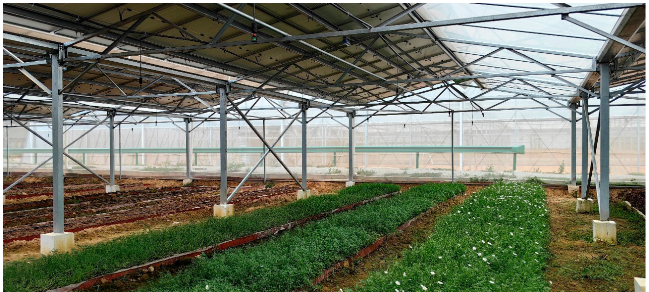
Figure 3. A real picture of the zigzag photovoltaic greenhouse.
