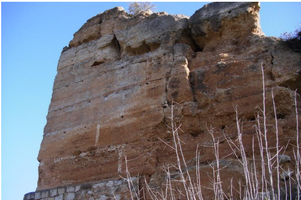
Figure 6. Detail of simulated ashlar stone masonry, in a rammed earth fortification.
