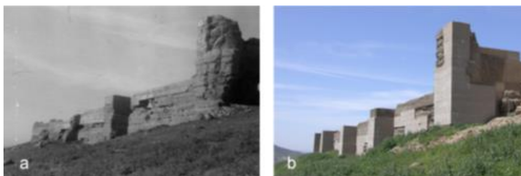
Figure 10. Recovery of volumes in a military rammed earth fortress to avoid collapse (Reina, Spain): a) before intervention; b) after intervention [31].
