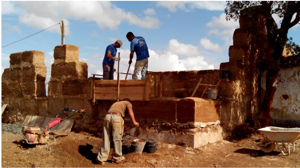
Figure 1. Example of civil rammed earth being produced in Santiago do Cacém, Portugal.
