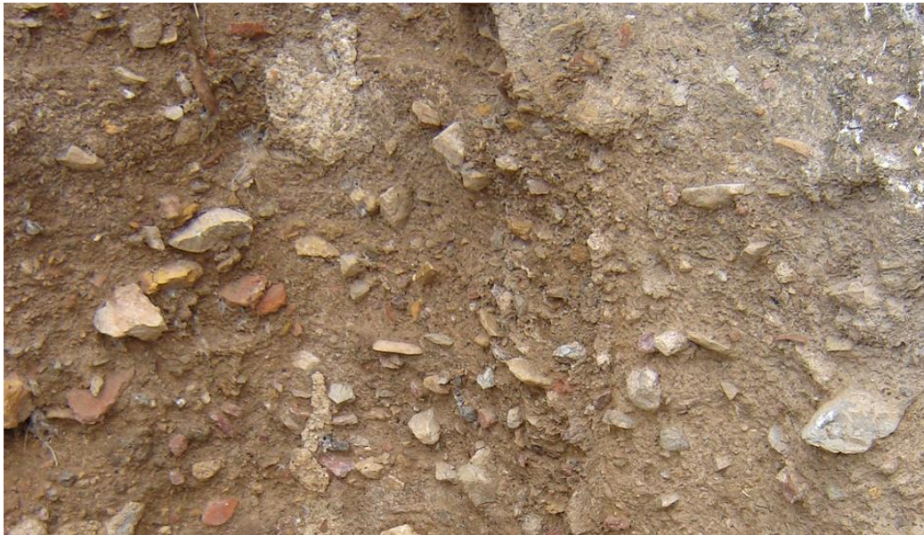
Figure 5. Detail of crushed red ceramic and medium size stones added to earth, in a rammed earth fortification.
