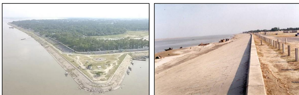
Figure 2. Sirajganj hard point along with the revetment (Source: Google image, and [7]).
