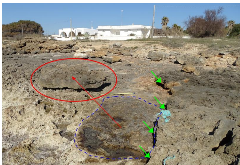
Figure A7. Mancaversa site; the MAa boulder lying about 4.5 m from its initial position (in the foreground); rock joints are indicated by green arrows (see text).
