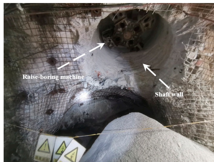
Figure 3. An ore-pass by raise-boring machine.
