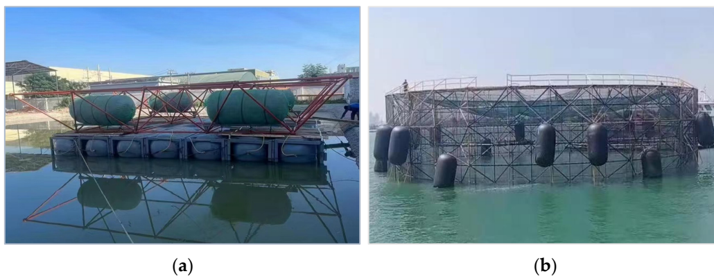
Figure 1. Steel grid structure with bolted ball joint: (a) Floating platform; (b) Deep-sea fish cage.
