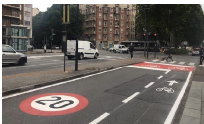
Figure 2. Controviali in Turin with bike priority and "case avanzate" in front of each traffic light.
