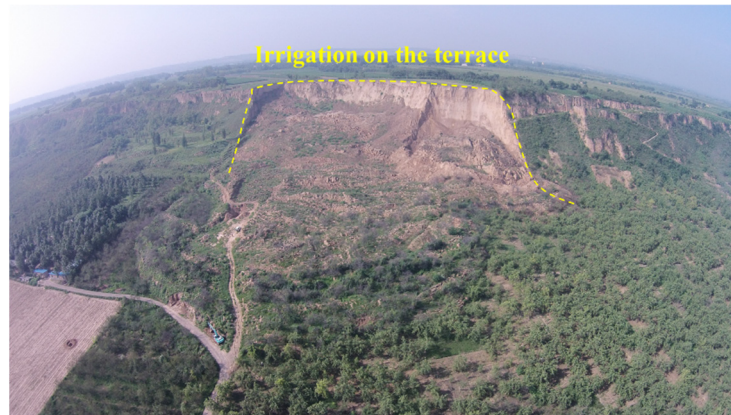
Figure 1. Photo of a typical landslide on the Heifangtai terrace due to irrigation, Gansu Province, China.
