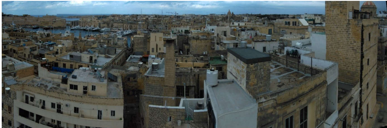
Figure 3. Different floor elevations and wall partitions in Senglea, which cause a drastic effect on generation
