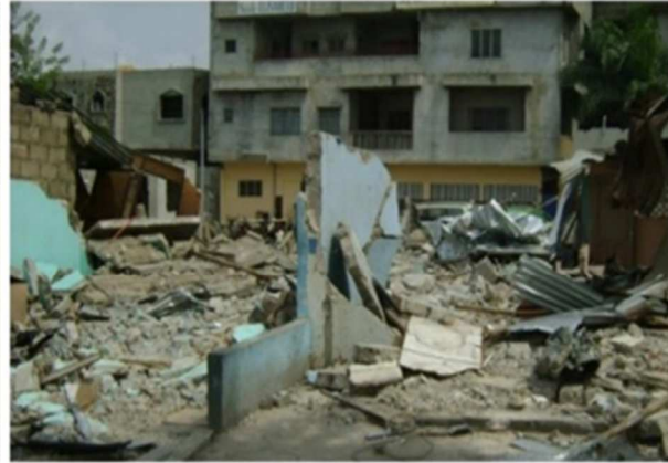
Figure 8: House demolition under justice decision in Tokan District, Abomey-Calavi( 2021)
