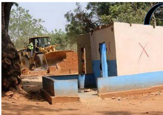
Figure 5: Loss of housing in Fidjrosse District, Cotonou (2018)
