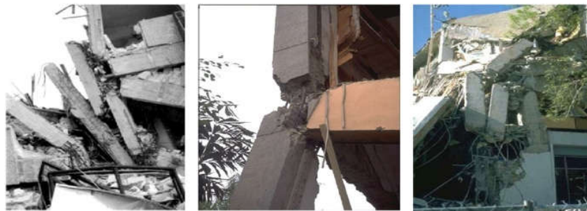
Figure 1. Partial collapse of buildings documented during large damaging earthquakes: from left to right: 1999 Izmit earthquake in Turkey, 1999 Chi-Chi earthquake in Taiwan, and 1994 Northridge earthquake in the USA.
