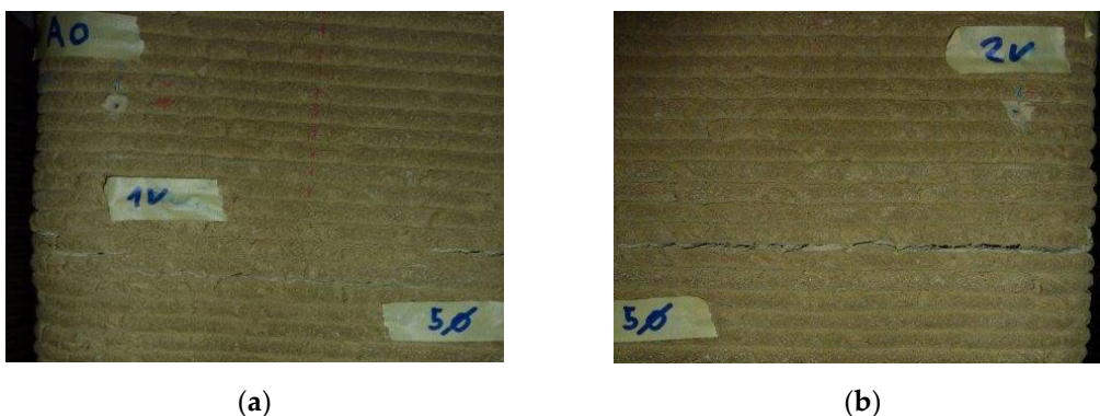
Figure 11. Details of the detachments between the horizontal layers of the side to the left of the operator: (a) Left detachment, which reaches edge 1; (b) Right detachment, which reaches edge 2.
