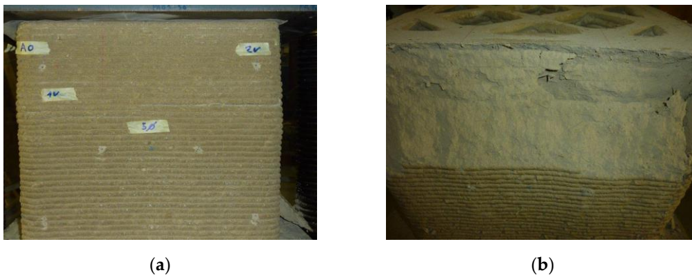
Figure 10. Failure mechanisms on the two short sides: (a) Side located to the left of the operator, extending between edge 1 (left) and edge 2 (right); (b) Side located to the right of the operator, extending between edge 3 (left) and edge 4 (right).
