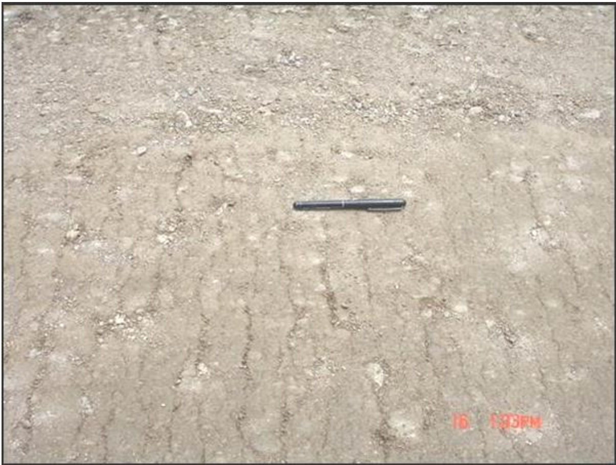
Figure 55. Appearance of small racking after roller compaction as an indication of moisture conditions that are too low for good compaction
