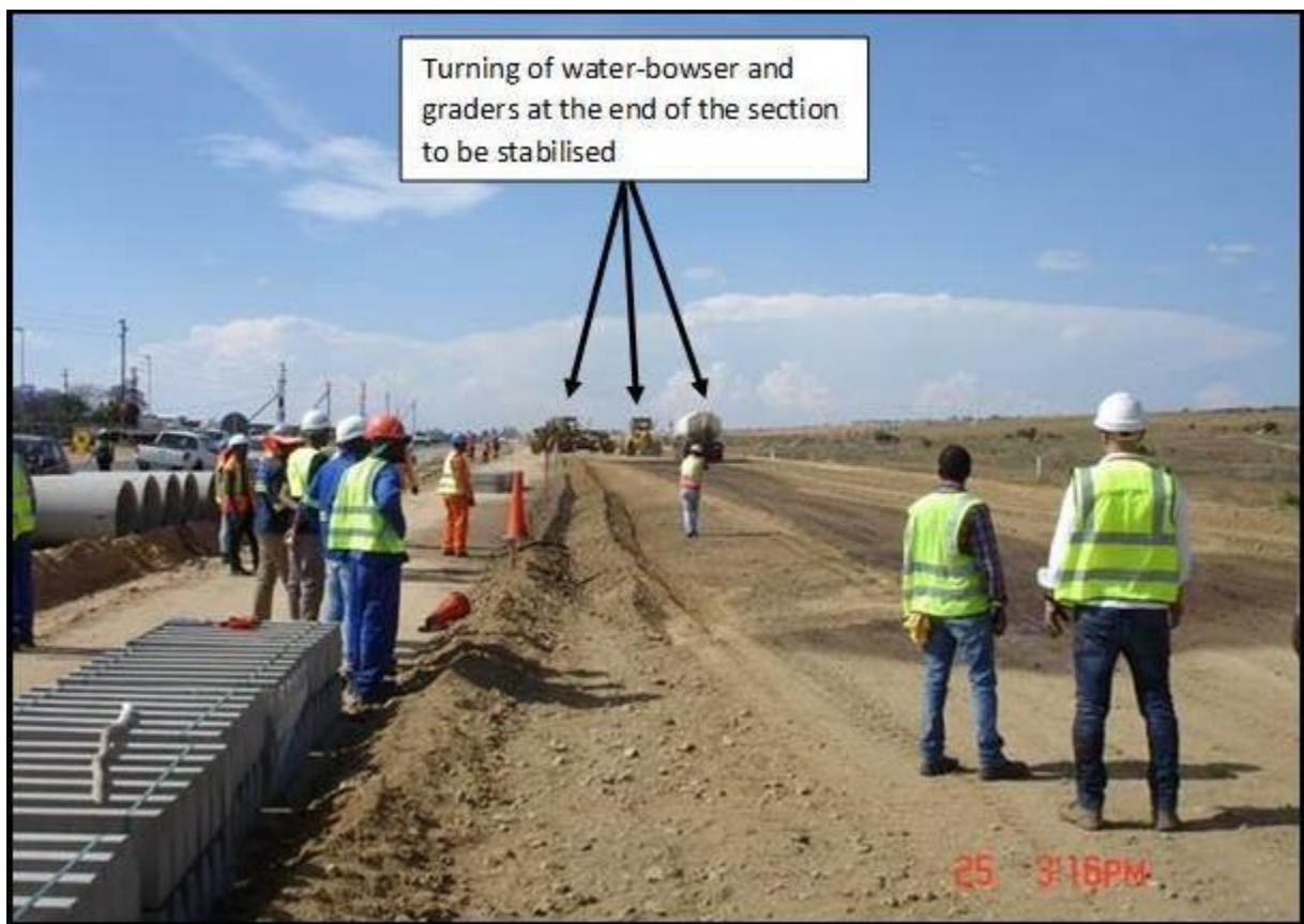
Figure 35. Turning of water-bowser and mixing graders at the end to the construction section, resulting in a longer construction time
