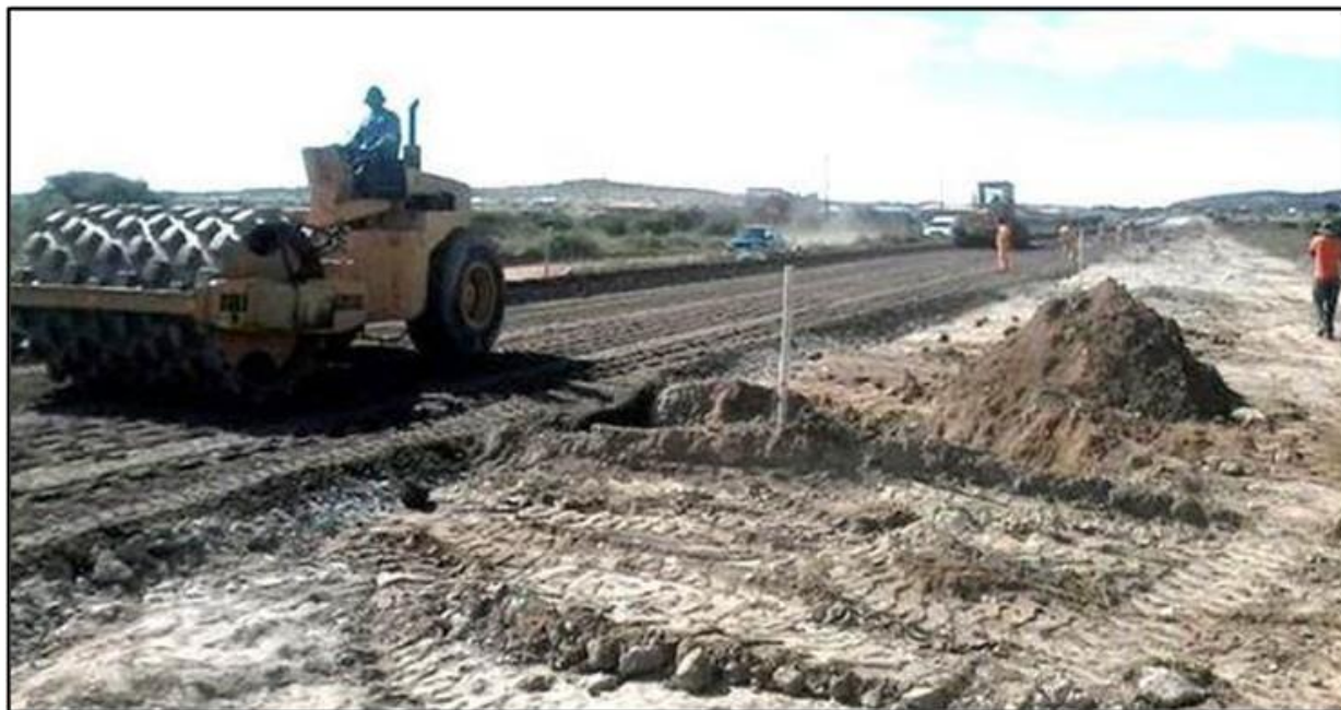
Figure 44. Compaction and cutting of final layer levels
