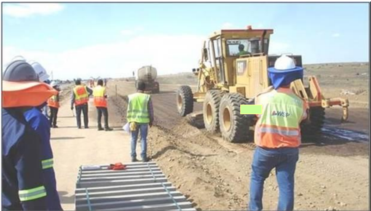
Figure 33. The water bowser is closely followed by graders that are mixing the NME stabilising agent dissolved in the construction water through the whole depth of the layer
