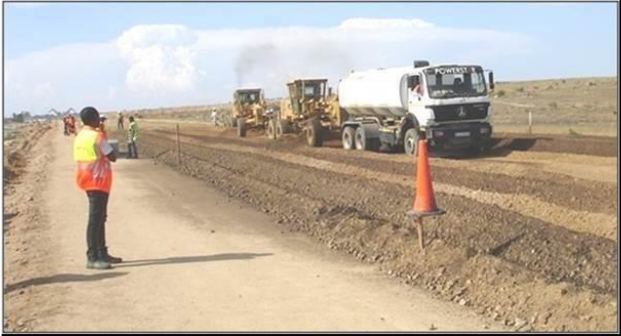
Figure 34. The spraying and mixing continue up and down over the whole width of the layer until the required stabilising agent is spread and mixed over the length, width and depth of the pavement layer
