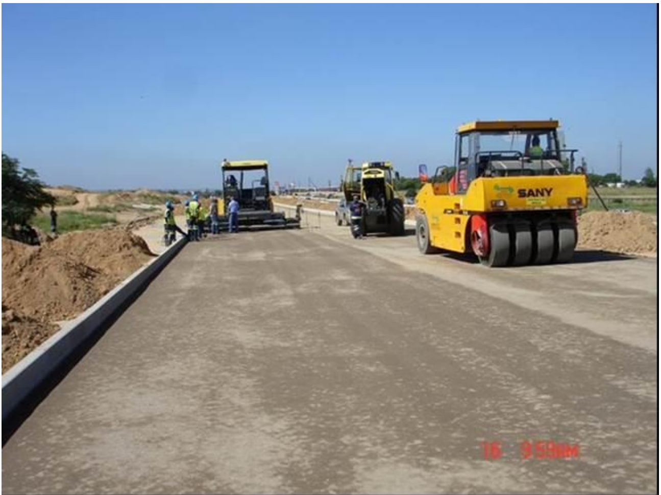
Figure 16. Placing of the 150 mm anionic NME stabilised base layer - note the quickness to which the layer is drying out
