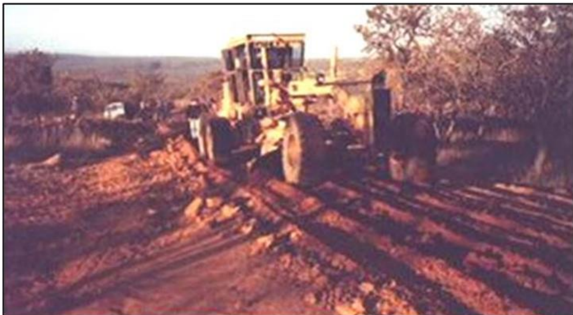
Figure 48. Ripping of layer to create layer depth exposure for ease of application of construction water diluted anionic NME stabilising agent
