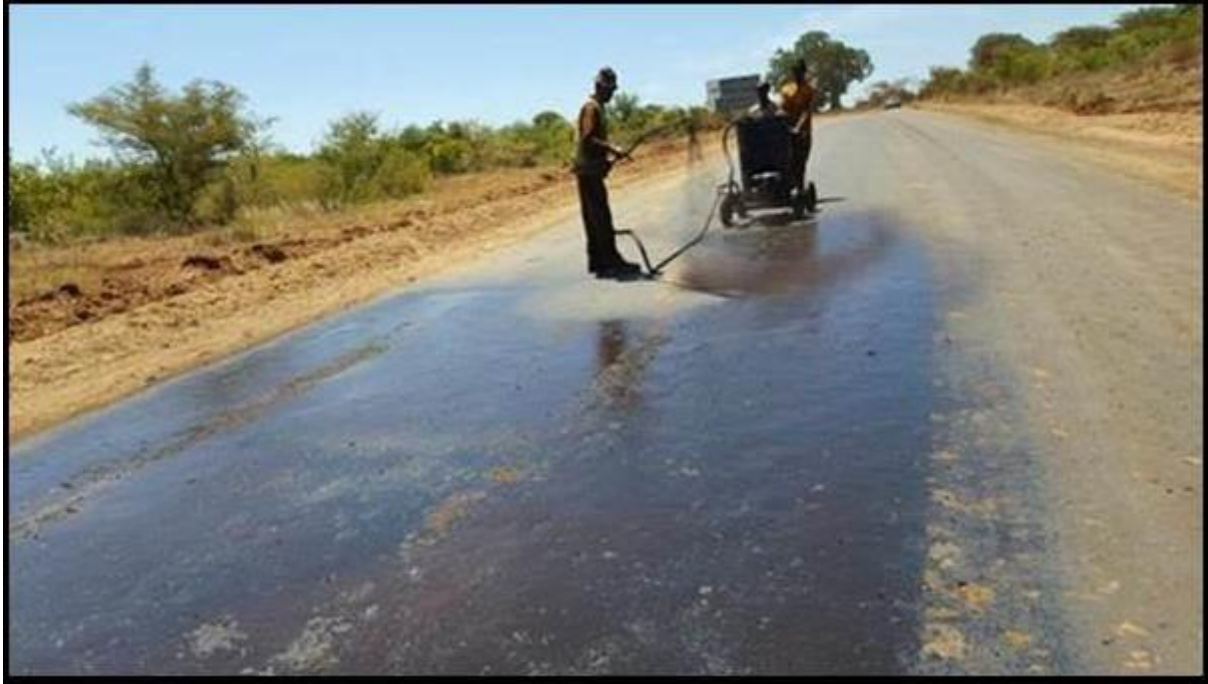
Figure 29. Hand application of a quick drying anionic diluted NME prime to protect the surfacing before application of the surfacing
