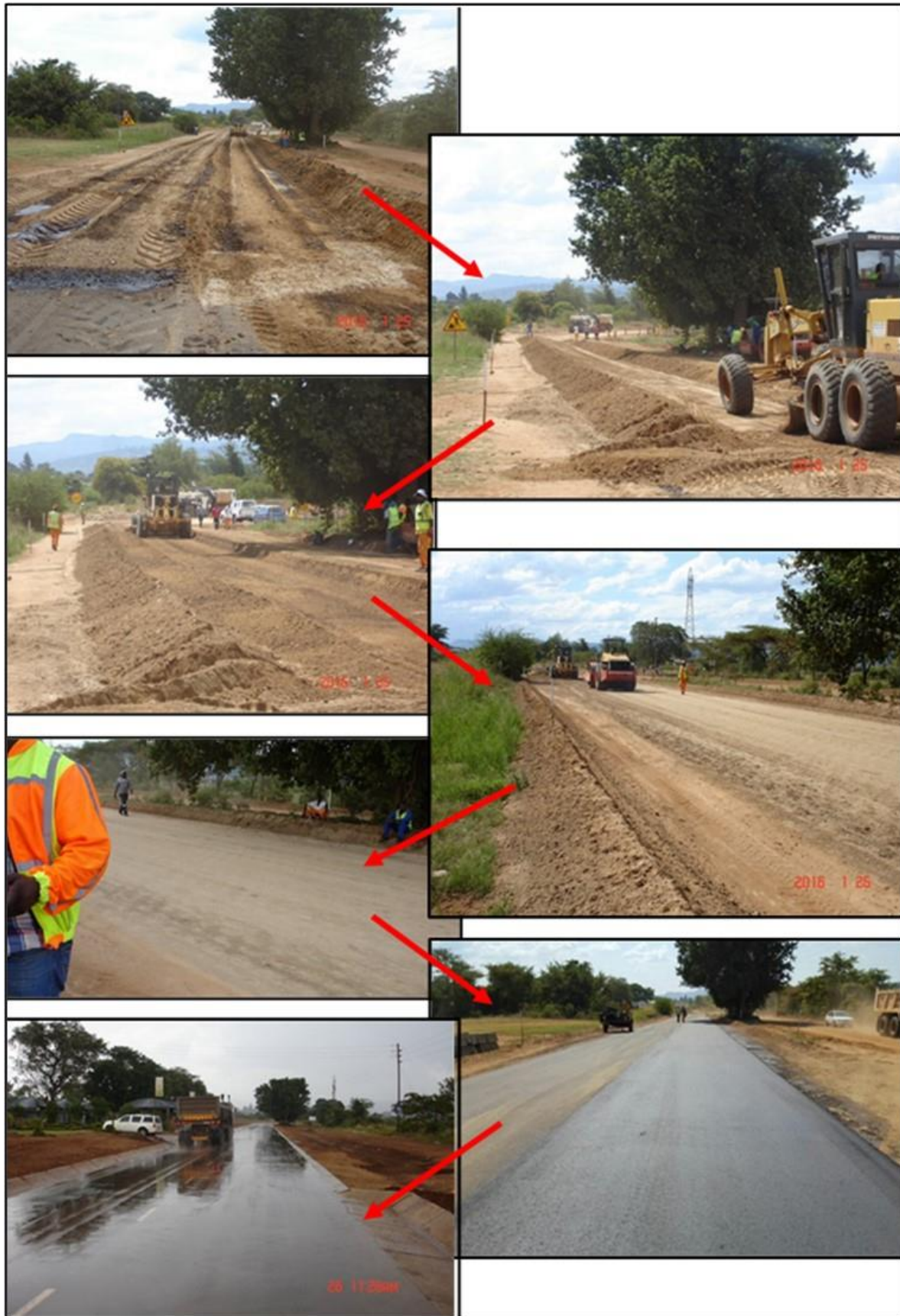
Figure 60. Resolving the uneven distribution of the NME stabilising agent through the remixing of the road pavement layer using conventional equipment.
