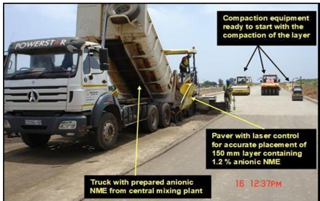
Figure 12. Delivery of anionic NME mix to site for the placement of the 150 mm base using a high accuracy paver
