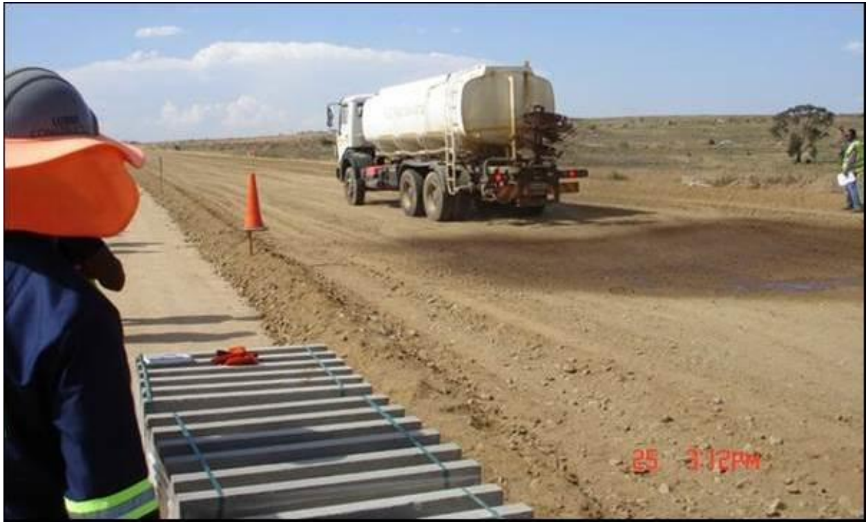
Figure 32. The sub-base granular material is spread along the section to be stabilised and compacted allowing for the compaction factor – the water-bowser containing the anionic NME pre-mixed with the required construction water is ready to start with the mixing process
