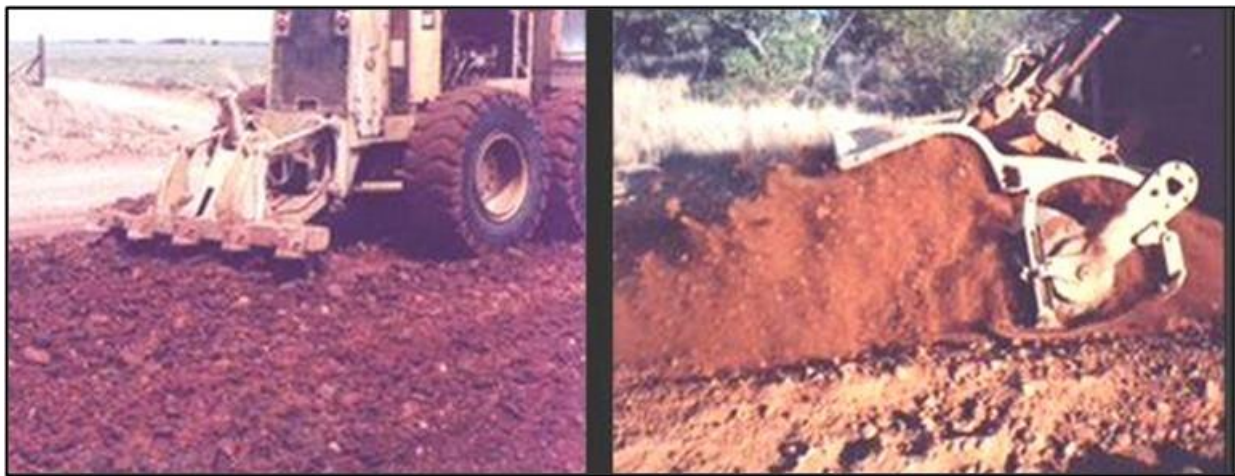
Figure 47. Ripping by grader and scarifying of in-situ material using a rotavator to loosen material to the required depth and expose oversized material for removal by hand
