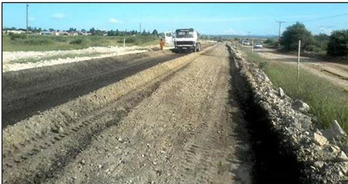
Figure 42. Water-bowser with construction water and anionic NME stabilising agent
