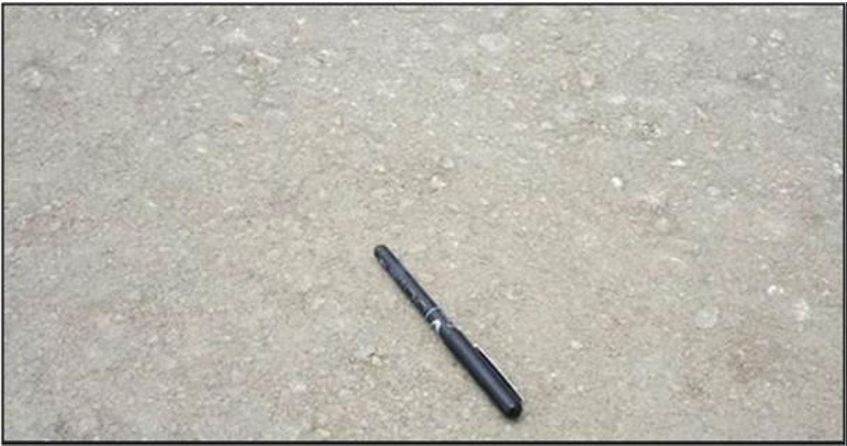
Figure 18. Final surfacing of the base-layer of the highway constructed with a 1,2 % anionic NME stabilising agent (~ 0.7 % residual bitumen) which was mixed in a central mixing plant and laid by paver to a tolerance of 2 mm before any additional protective material was added
