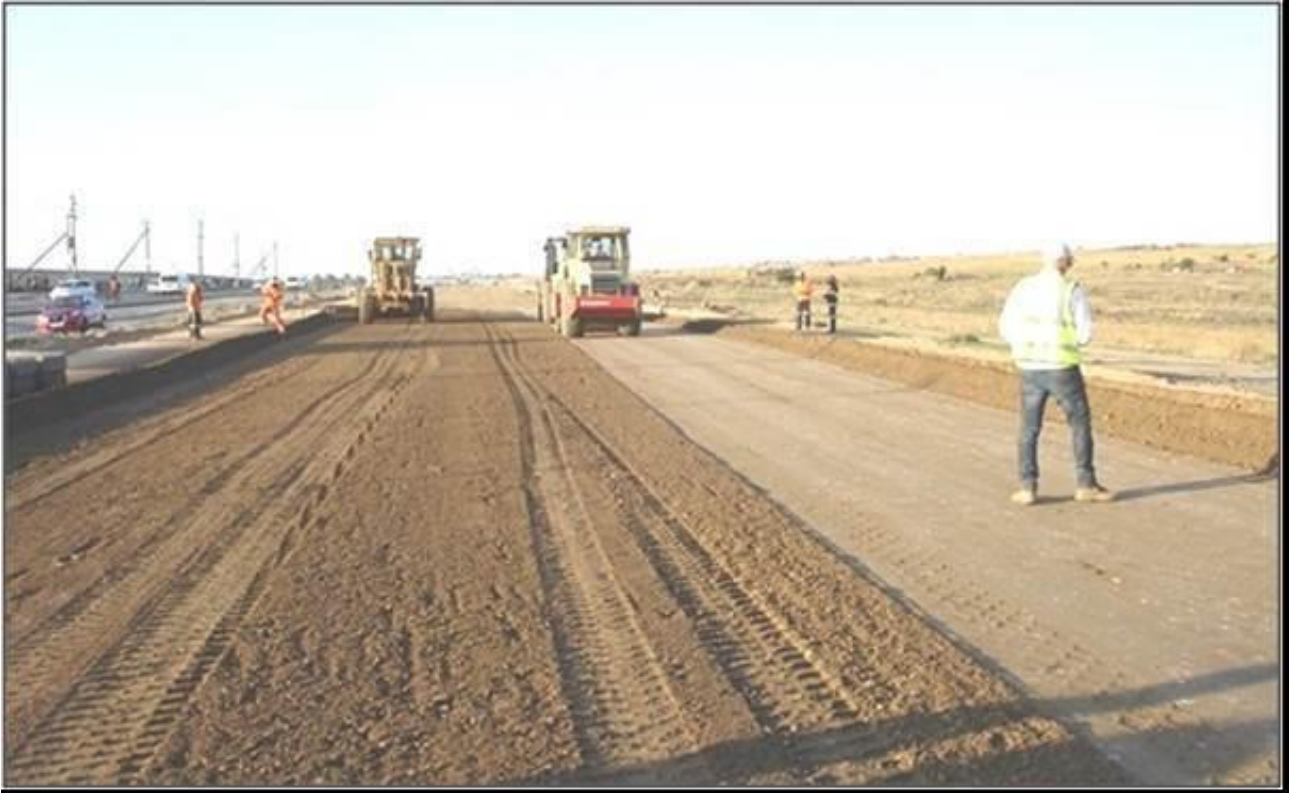
Figure 36. Shaping and compaction of the anionic NME stabilised layer (0.7 % NME with G5/6 quality granular material)
