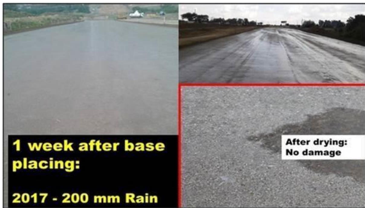
Figure 20. The unprotected base-layer (Figure 18) stabilised with 1,2 % anionic NME, was severely tested when subjected to 200 mm of rain the week after placement with no damage to the layer – a practical proof of the water-resistant (hydrophobic) nature of the anionic NME stabilising agent used for the stabilisation of the G5/G6 (refer Figure 1) granular material
