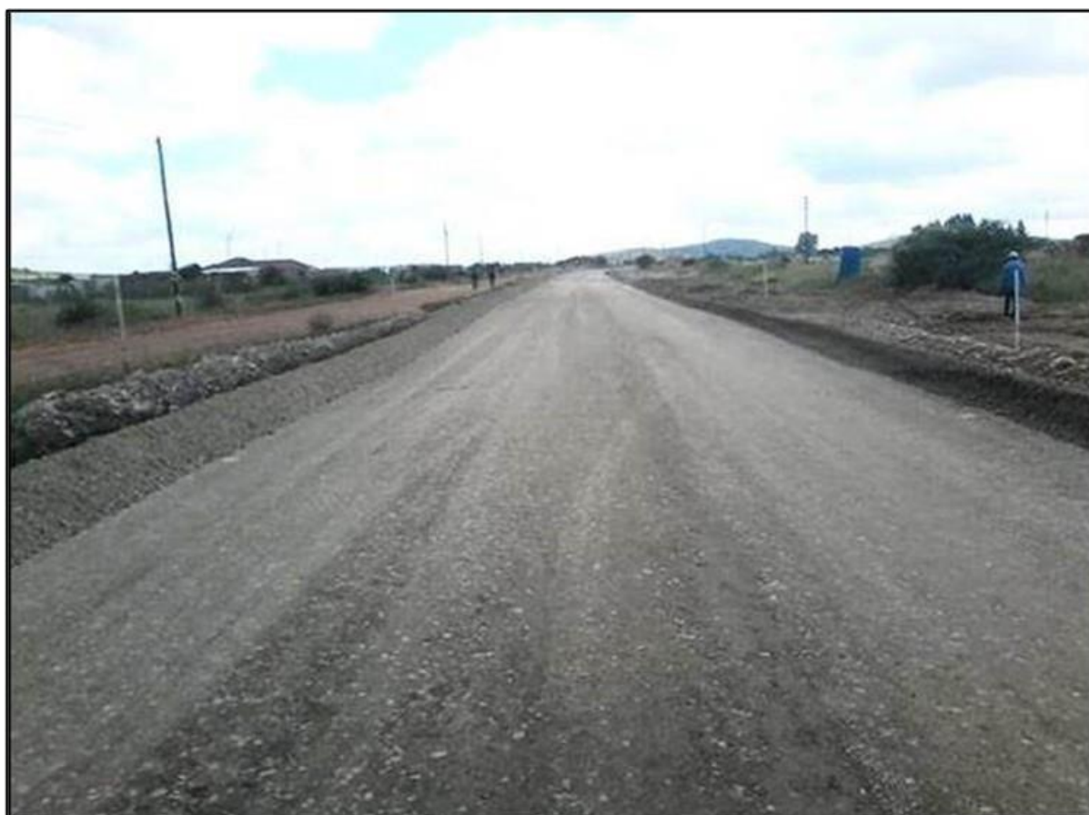
Figure 45. Condition of the compacted layer prior to applying a tack-coat and surfacing
