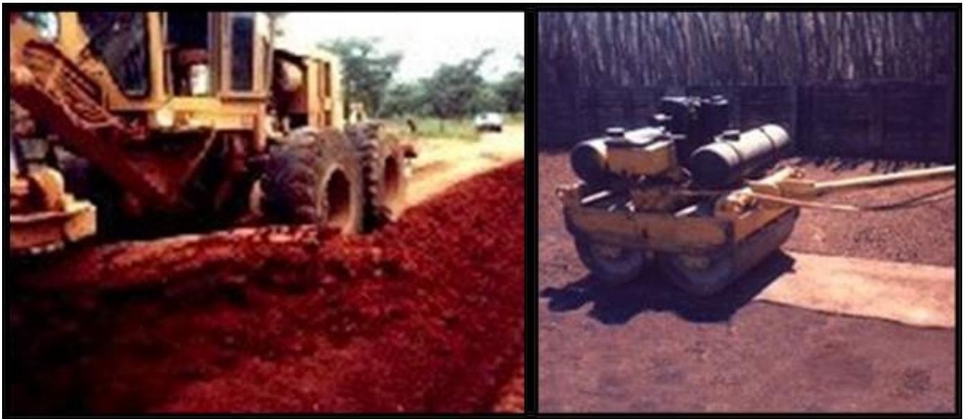
Figure 50. Mixing by grader and compaction using hand operating compaction equipment
