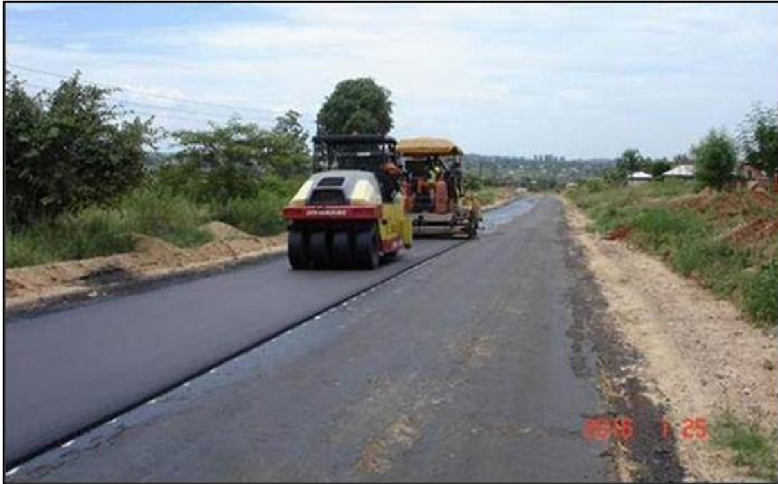
Figure 31. Surfacing of the rehabilitated urban road (Figures 24 to 29) after two months of trafficking during the summer holidays
