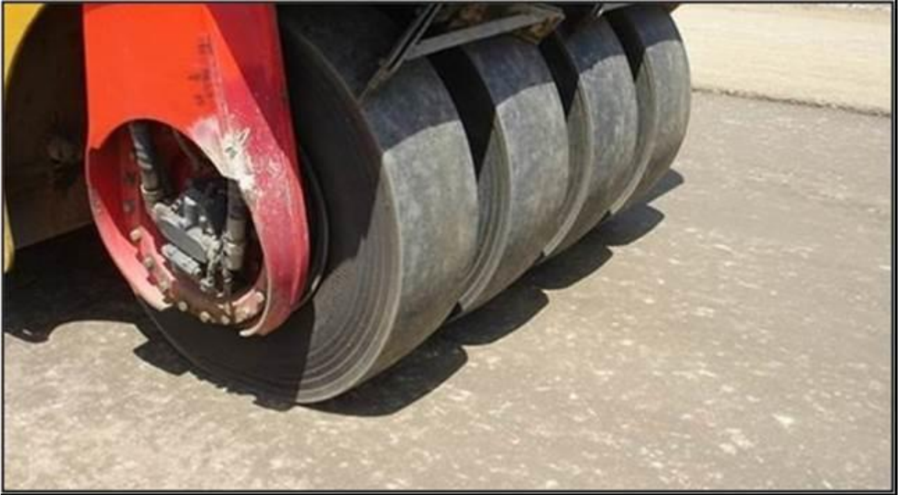
Figure 15. Final compaction of the base-layer constructed with a 1.2 % anionic NME stabilising agent, mixed at a central batching plant and placed with a paver
