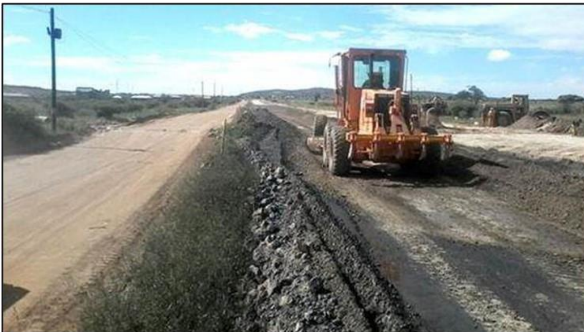
Figure 43. Single grader used for mixing of the anionic stabilising agent pre-mixed within the construction water
