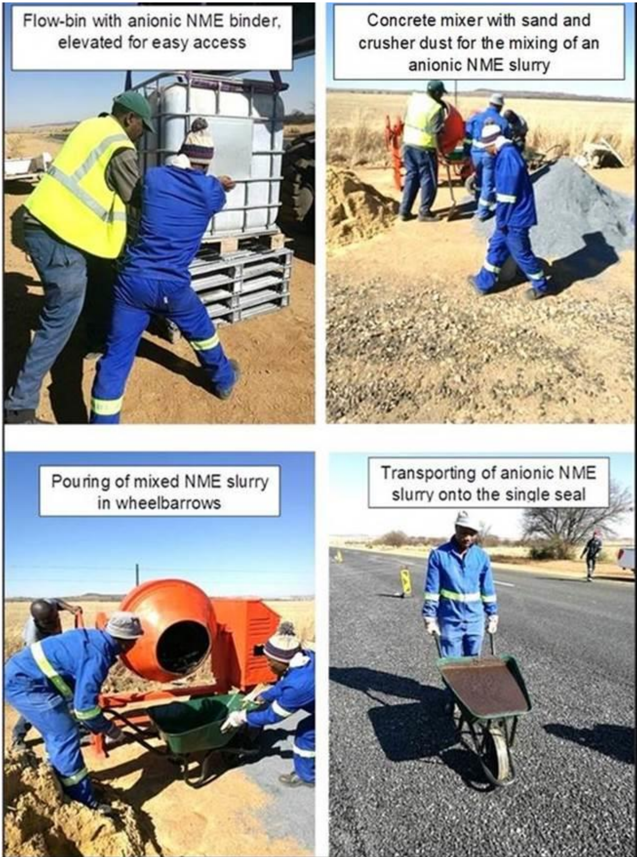
Figure 52. Labour-intensive road-side manufacturing of the slurry mix for a modified Cape seal using an anionic NME binder
