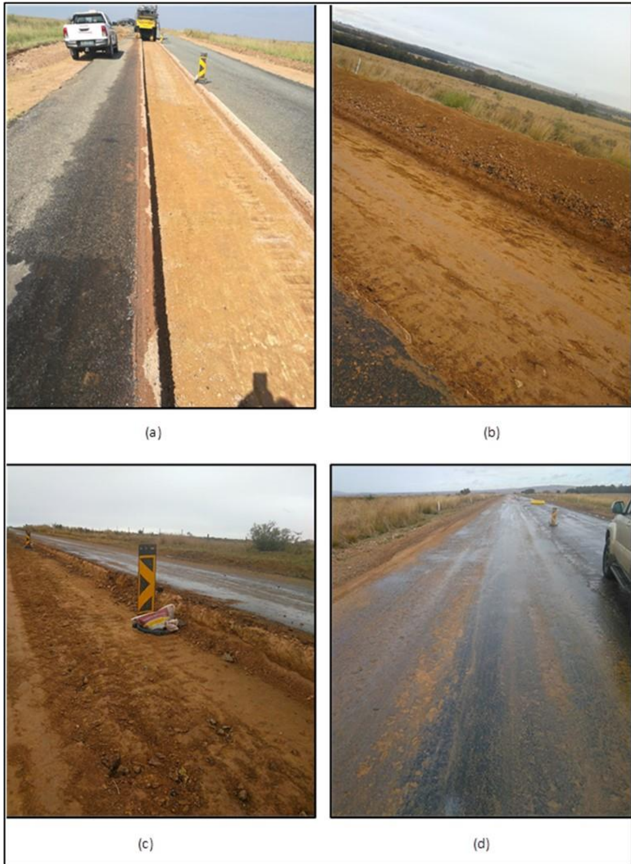
Figure 63. (a) Milling of existing base and sub-base layers to be stabilised using an anionic NME stabilising agent (b) stockpiling of material next to the road (c) showing depth of milling and new road-bed to be compacted and (d) showing the reintroduced sub-base and base separately stabilised using an anionic stabilising agent
