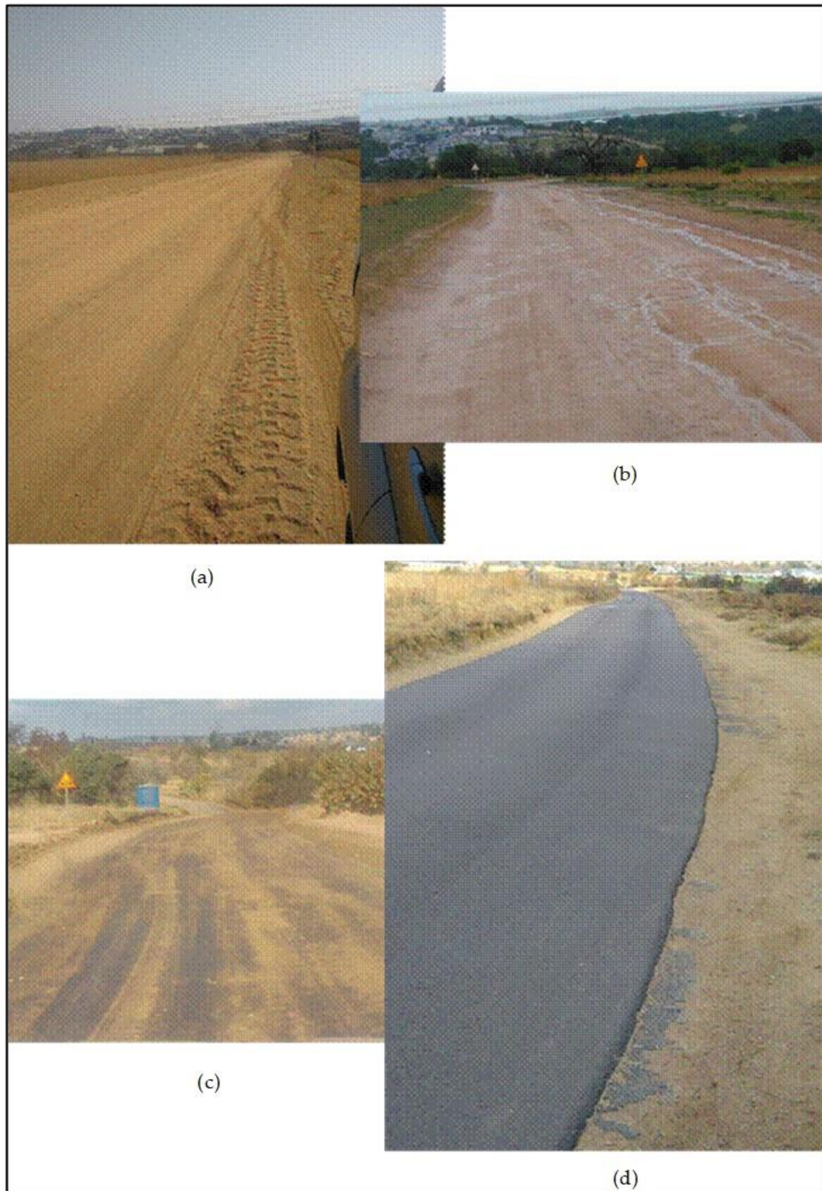
Figure 54. Upgrading of a local access road with (a) and (b) showing the sandy/slippy/muddy conditions prior to upgrading; (c) 100 mm in-situ stabilisation with an anionic NME stabilising agent and (d) with an ultra-thin fine-graded asphalt surfacing
