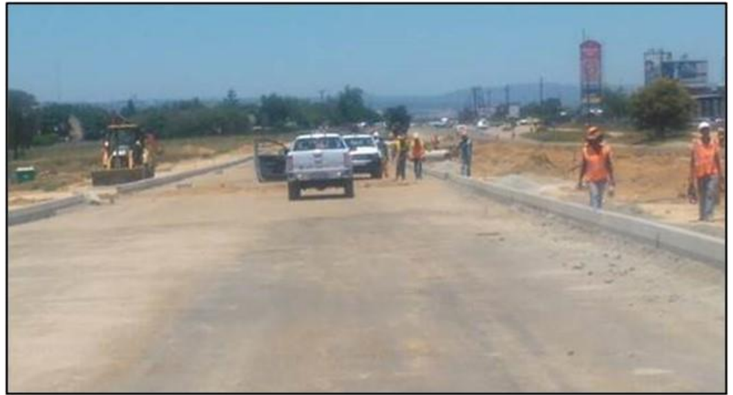
Figure 11. Prepared sub-base with installed curbs for the inter-city freeway under construction
