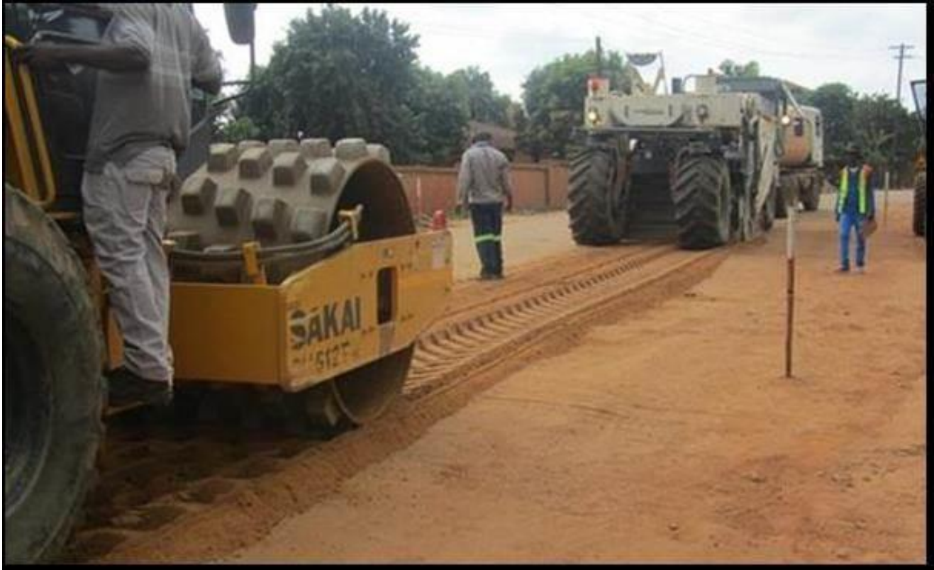
Figure 27. Construction train for the in-situ recycling and NME stabilisation of the severely distressed road.
