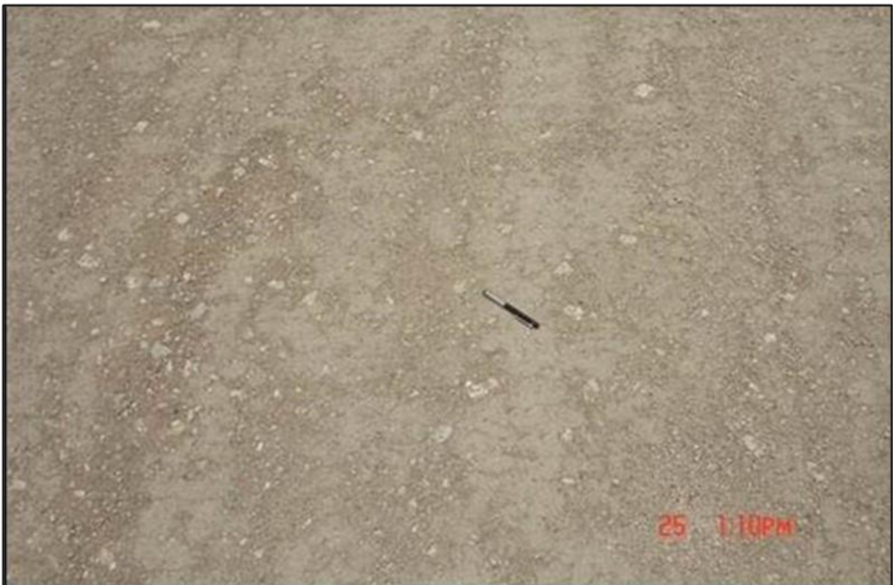
Figure 41. Close-up of the sub-base layer constructed with 0.7 % anionic NME stabilising agent, using conventional construction equipment and after being subjected to a considerable amount of rain – the hydrophobic efficiency of the organofunctional silane modification of the bitumen emulsion modification has shown effective in practice
