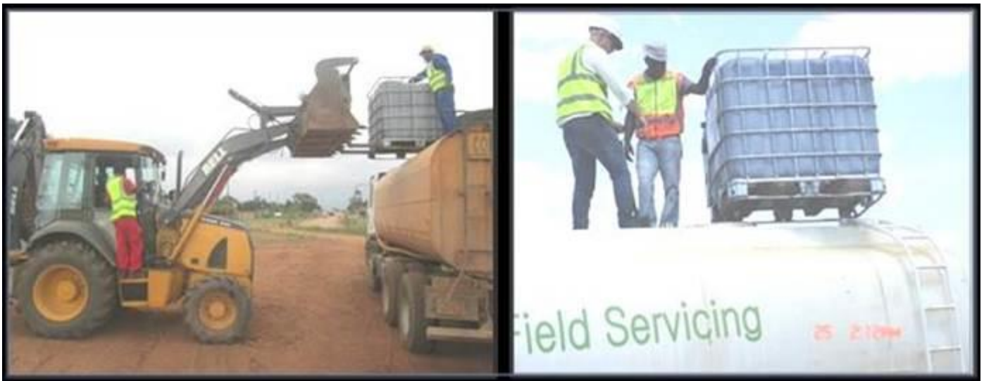
Figure 21. Using basic equipment and gravity to add the anionic stabilising to the construction water already in the water-bowser. The volume of water and that of the stabilising agent would have been calculated on the basis of the volume of granular material to be stabilised
