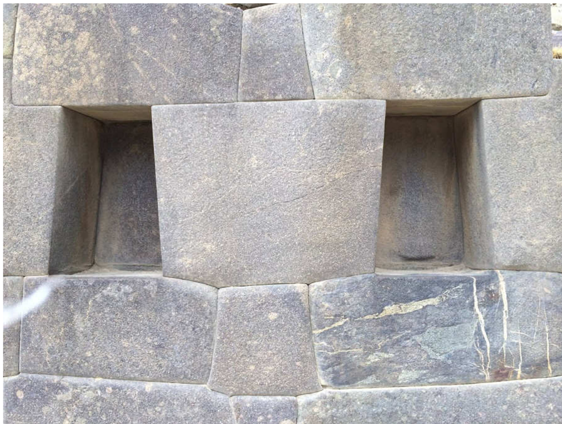
Photo. 11. Temple of Ten Niches, Ollantaytambo (A. Fuchs, 2008, sy-akka.de/wordpress). Pay attention to the symmetrical arrangement of the blocks in the masonry.
