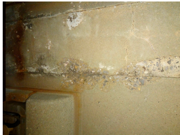
Figure 2. Cracking at wide and narrow joints
